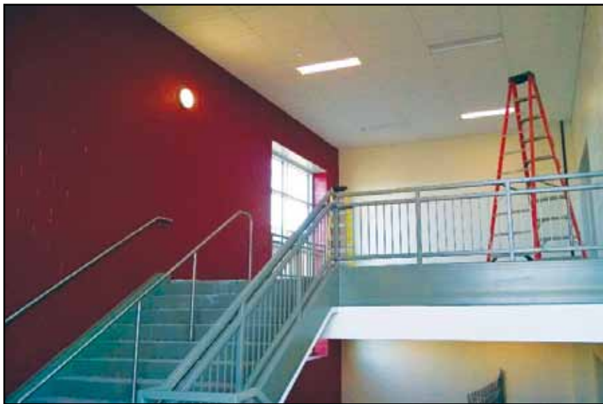
Phase three stair tower 98% complete
